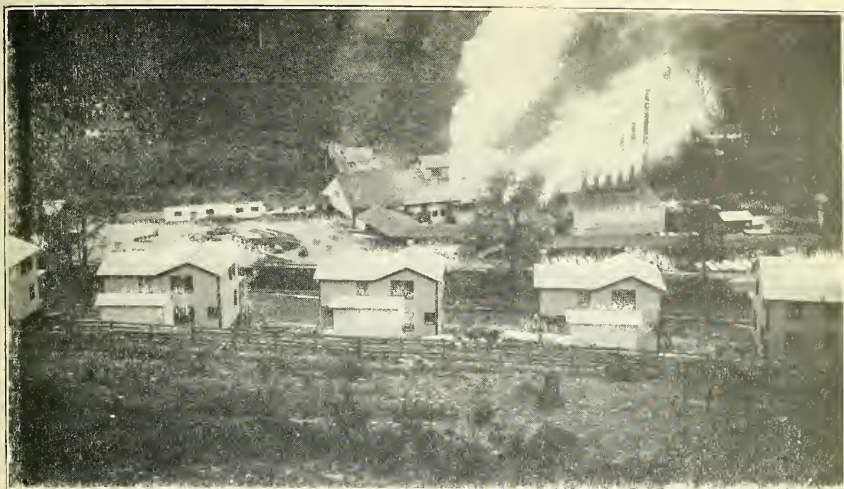
PLATE XXX (a).—Gauley Mill of Cherry River Boom and Lumber Company at Gauley Mills.
